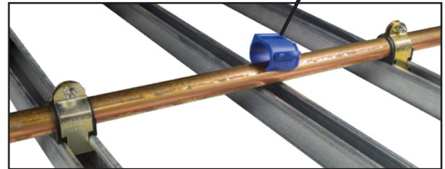
**Step 4:** Add Pipe Clamps and tighten the assembly.
